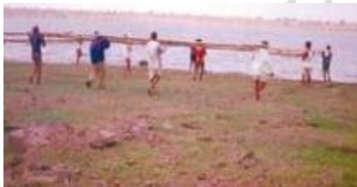
Four poles are used to make one long side of the rectangle. Two poles are placed on the ground with their tip portions overlapping to make their combined length at least 14.5 meters. Six such lengths are made for the two long sides and the central divider. Each long side and the central divider consist of two such 14.5-metre lengths placed parallel 35 cm
