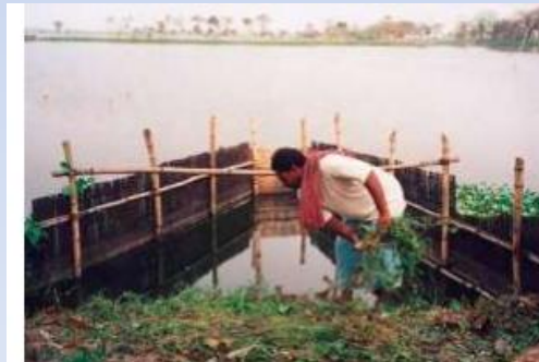
3. Bamboo sluice & dikes are repaired
