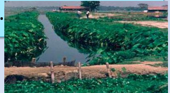
Allow sewage flow in pond through open channel
